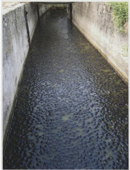
FIGURE 1. Site C is an abandoned agricultural ditch artificially filled with water by the landowners that acts as an ephemeral Spea intermontana breeding site. After a length of 6 m, sand berms are constructed in the ditch for amphibian entrance to and exit from the water. Photo credit: R Firman 2010.
