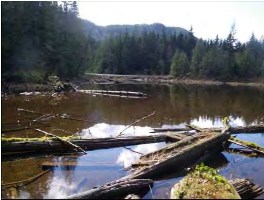
Photo K. Looking west at Lost Creek Road 4K East on March 31 st 2010.
