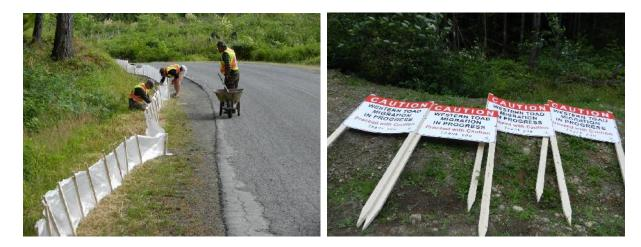
Figure 1. Directive fencing, pitfall traps, and educational signage installed along Barnjum and Riverbottom Roads near Wake Lake in Duncan to safely move dispersing toadlets across the road.
