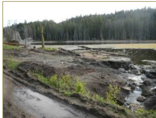
Disturbance to the shoreline and breeding habitat in Kane Valley associated with removal of an old dam structure, 24 May 2013.
