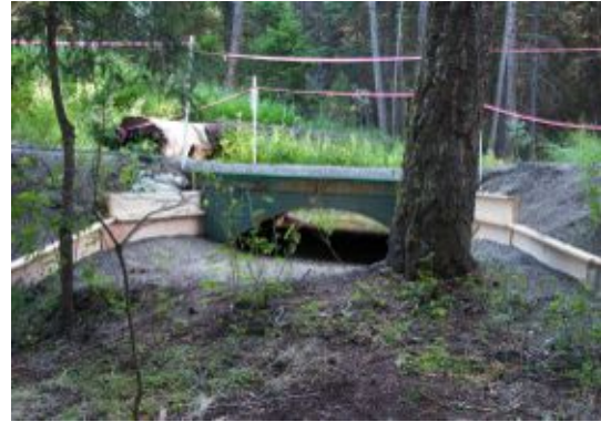
The underpass with funnel leading to the entrance.
