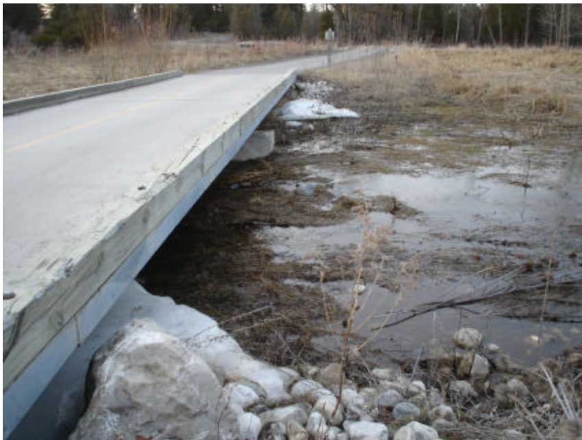
Figure 5: RIM Park: April 5, 2005. Herpetofauna pond and clearspan (Photo taken by author).
