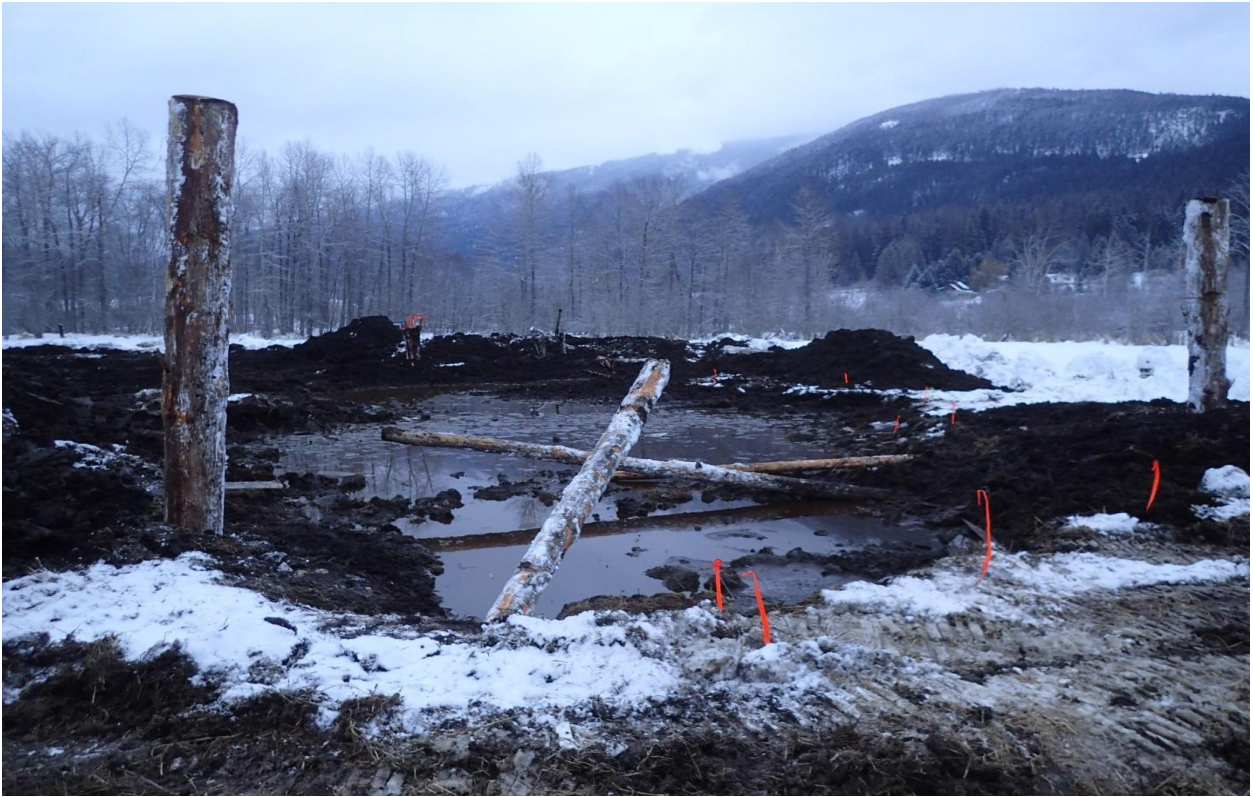
Figure 10. Posts and basking logs installed in the third wetland, January 2019.
