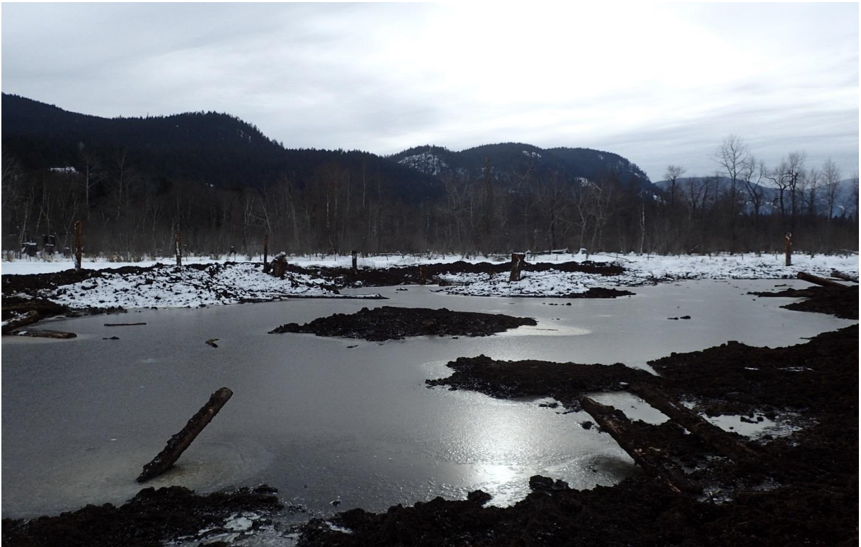
Figure 11. Wetland excavation completed, January 31, 2019.
