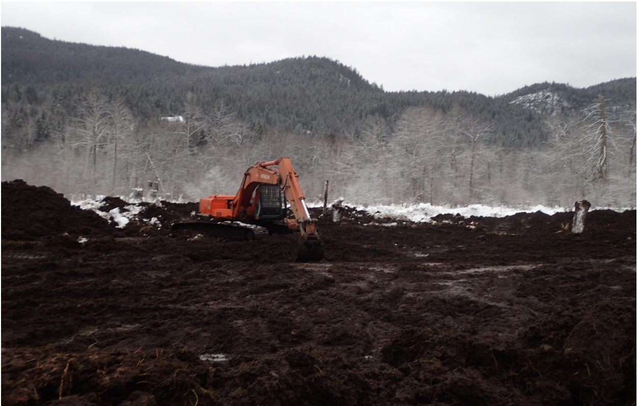
Figure 9. Excavating the third wetland, January 2019.
