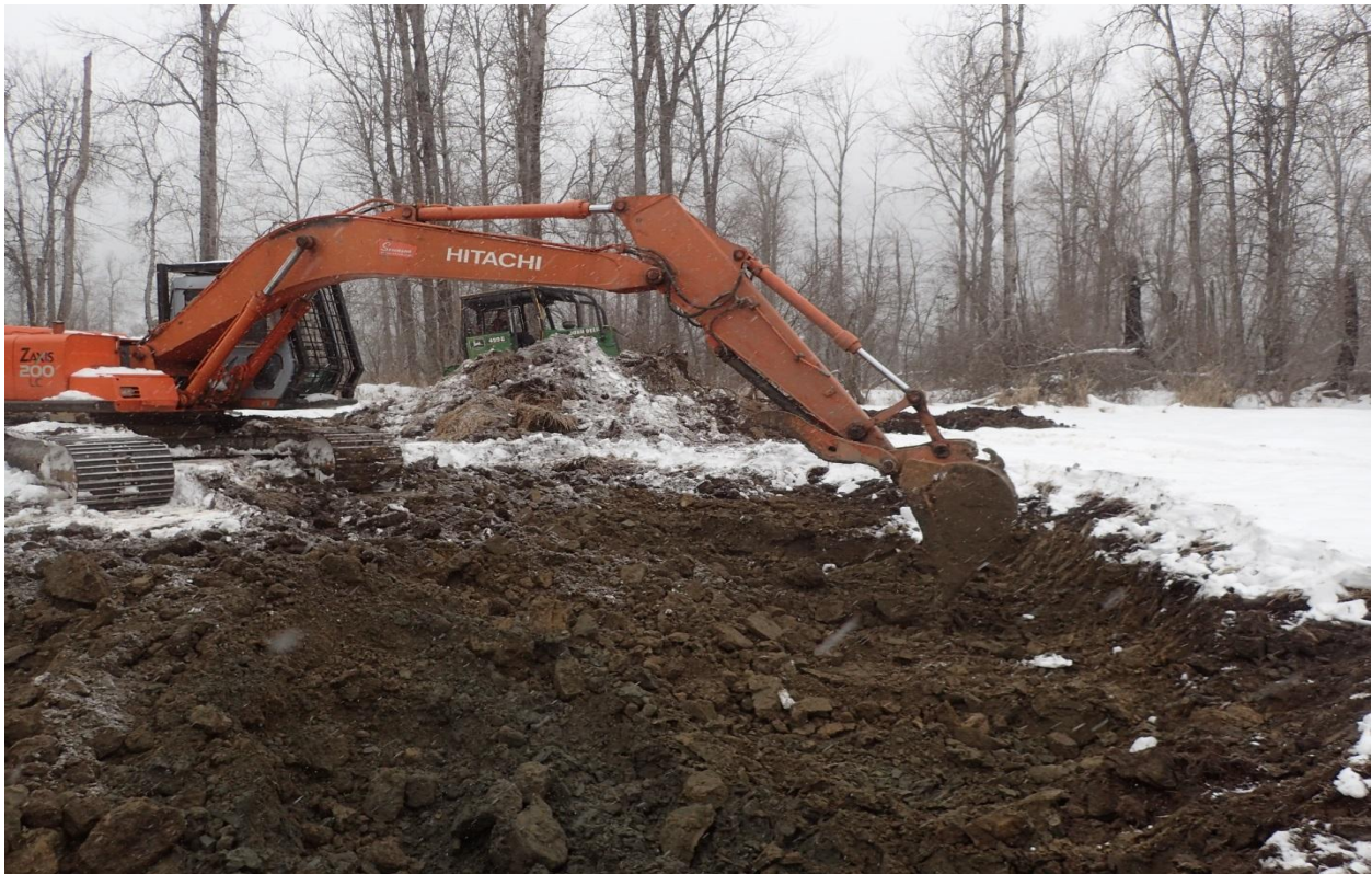
Figure 6. Excavating the first wetland, January 2019.
