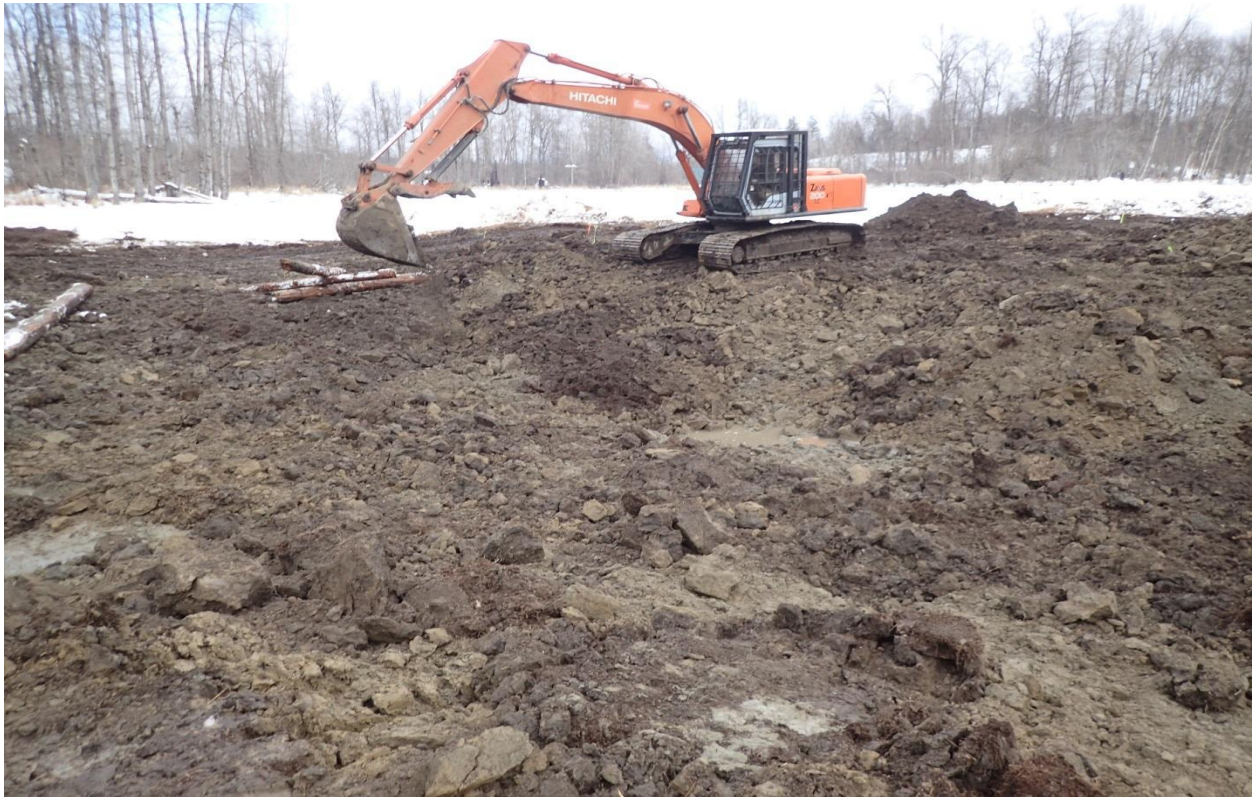
Figure 7. Excavating the second wetland, January 2019.
