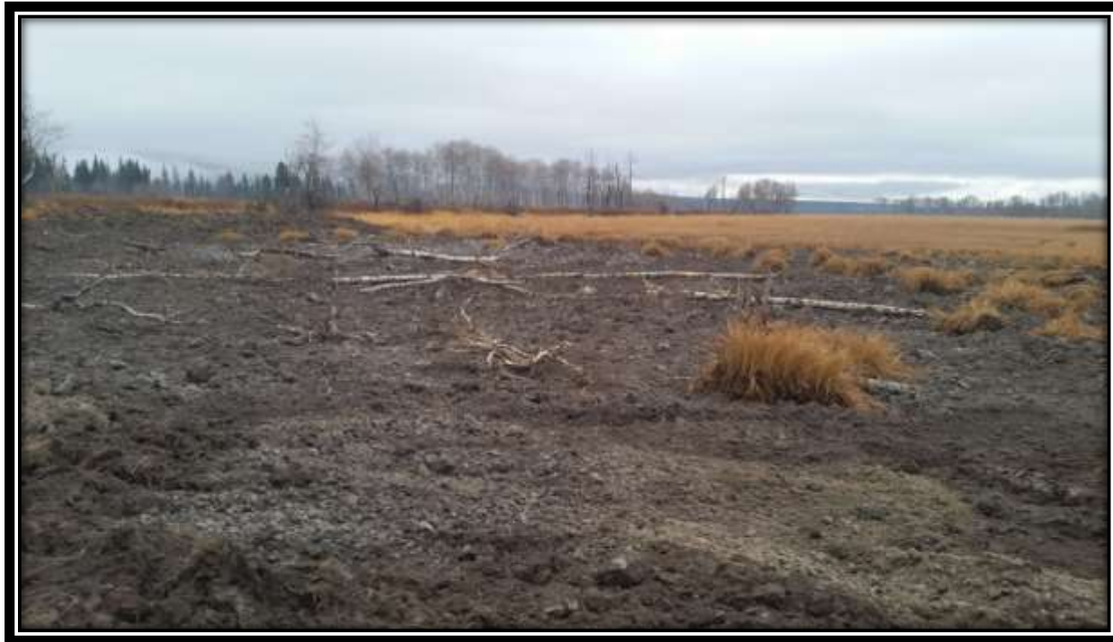
Photo 14: Woody Debris placed in the Shallow Wetlands
