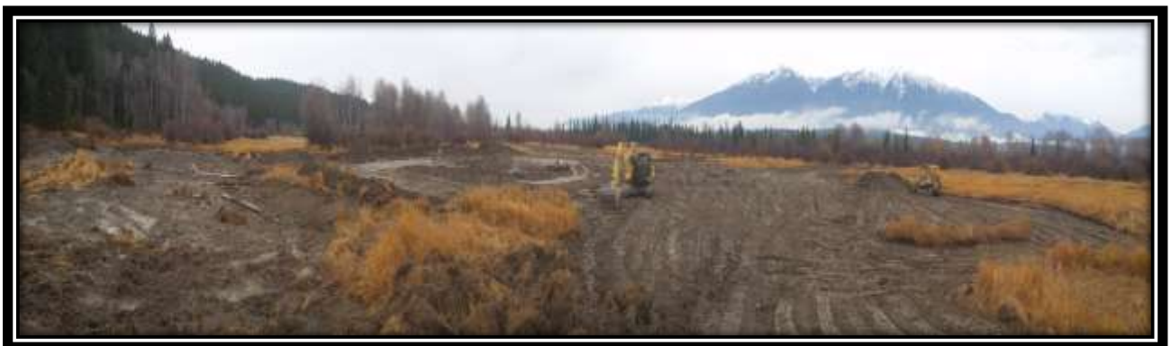
Photo 11: Completion of Shallow Wetlands and Mounds on Wetland Site 1
