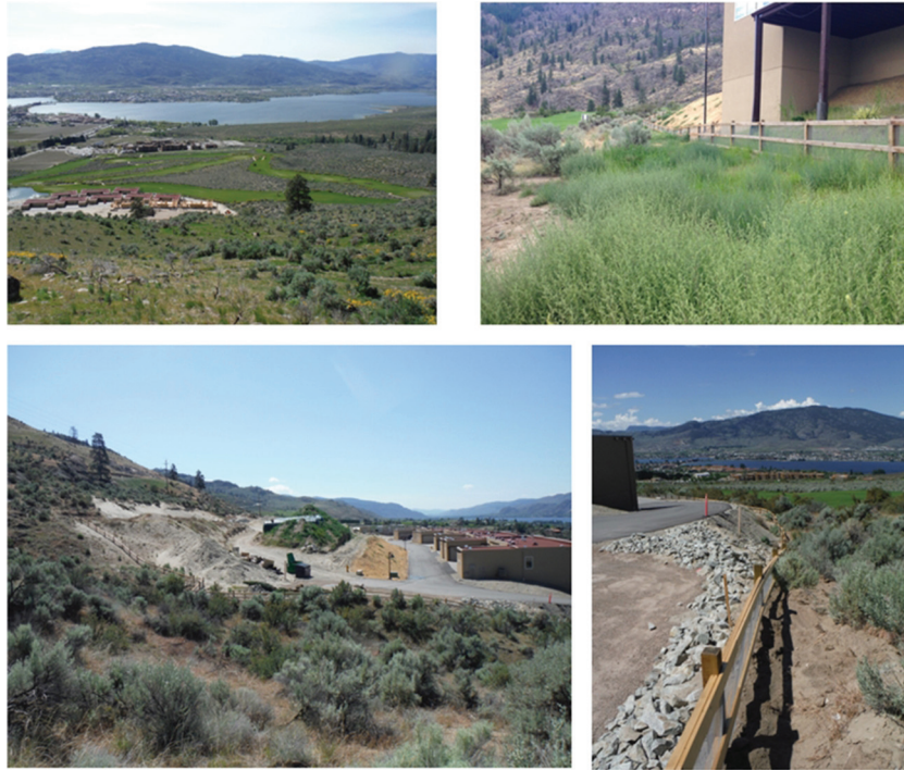
Fig. 2. Condominium community and construction with surrounding mitigative wooden snake fence structure. Colour version online.
