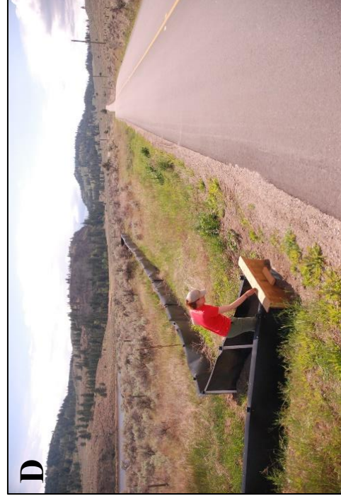
Figure 1.4. Examples of snake road mortality mitigation measures in the White Lake Basin, British Columbia, including A) a modified culvert equipped with a camera, with the entrance unaccompanied by fencing, B) a newly-installed semi-circular ecopassage equipped with a camera and fencing surrounding the entrance, and C & D) drift fencing positioned to funnel snakes into under-road ecopassages. (Photo credits: Karl Larsen)
