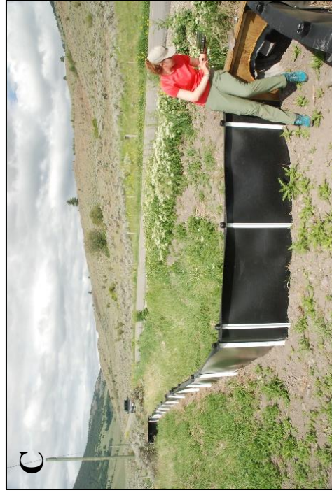
Figure 1.4. Examples of snake road mortality mitigation measures in the White Lake Basin, British Columbia, including A) a modified culvert equipped with a camera, with the entrance unaccompanied by fencing, B) a newly-installed semi-circular ecopassage equipped with a camera and fencing surrounding the entrance, and C & D) drift fencing positioned to funnel snakes into under-road ecopassages. (Photo credits: Karl Larsen)
